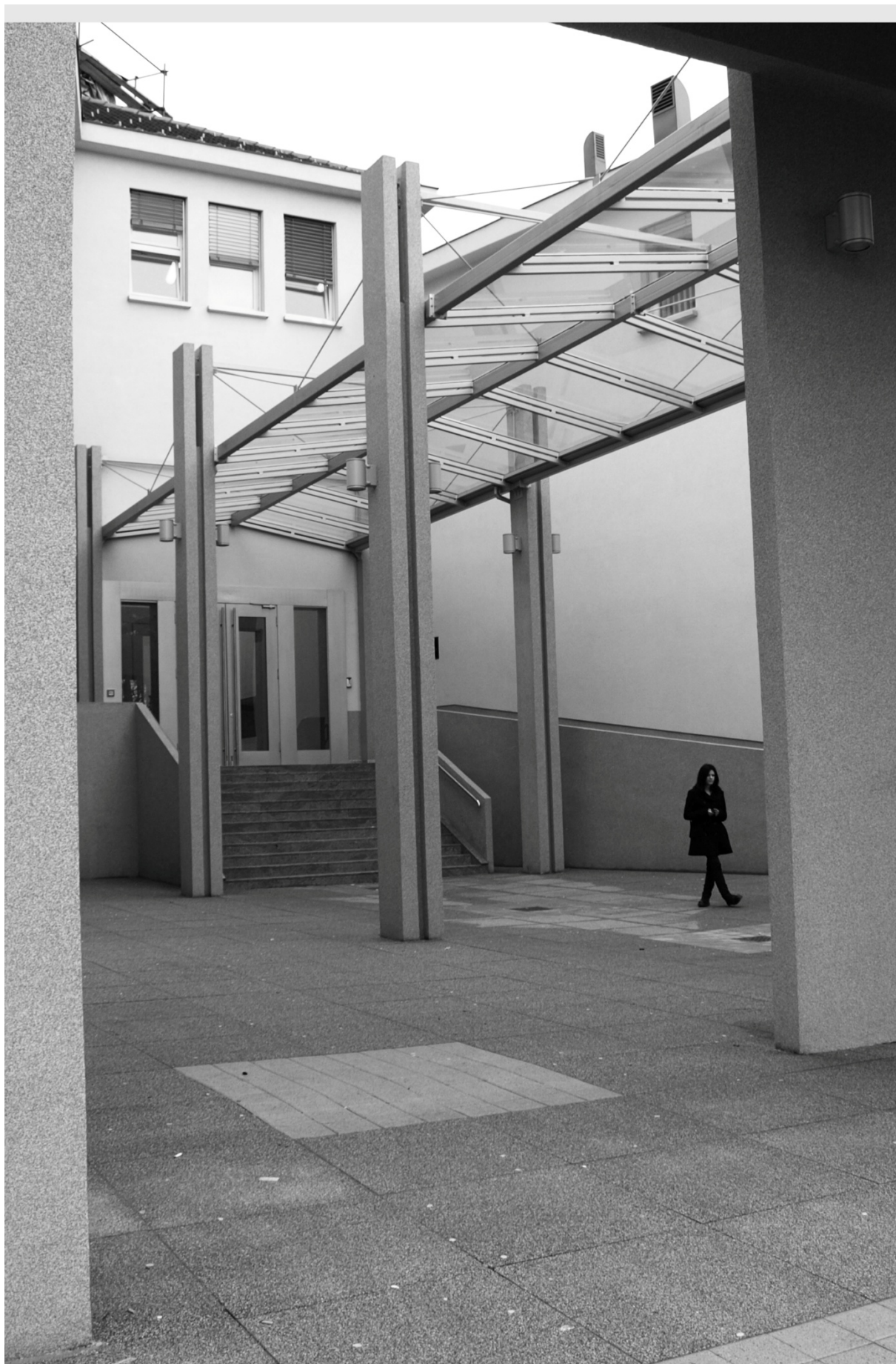
Photo 041. The new high school building / Nova zgrada Gimnazije
